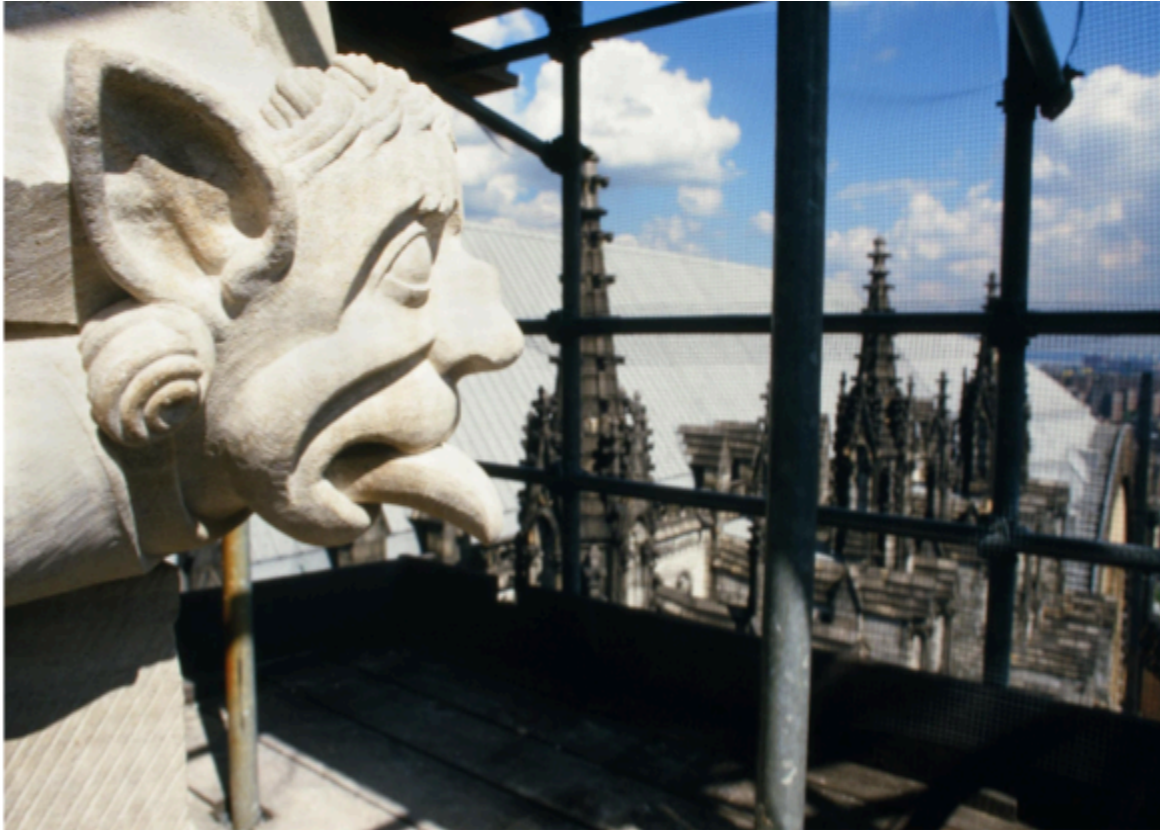
Carving in place atop tower. Photographer Robert F. Rodriguez
